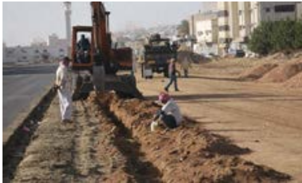
Continued completion of sewage connections in the city Buraidah
