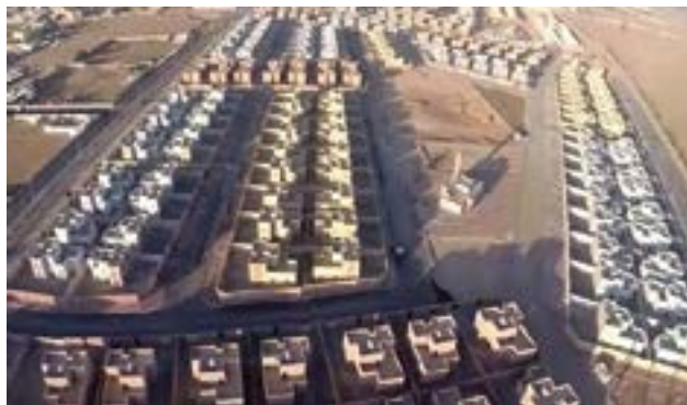
Shaqa housing Project in Buraidah
